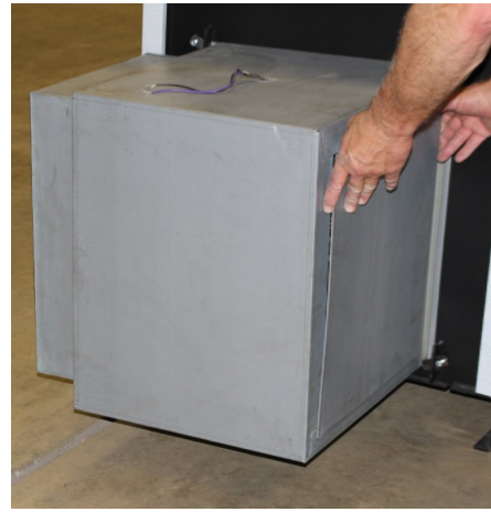
Installing Block Off Jacket
