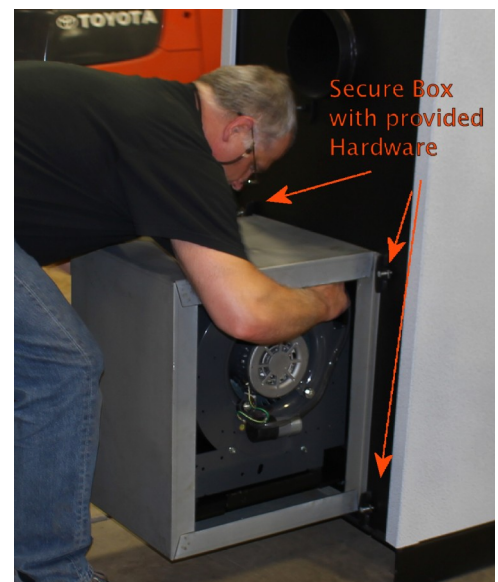
Securing Filter Box
