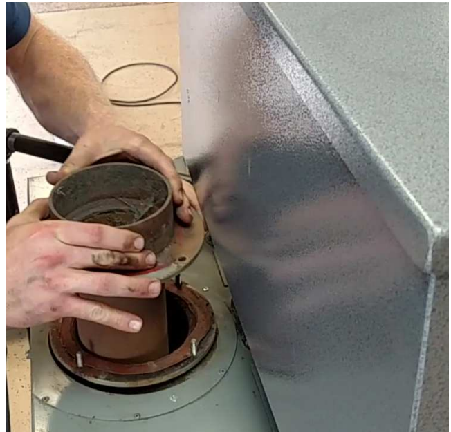
Lifting Out the Flue Tube Assembly
