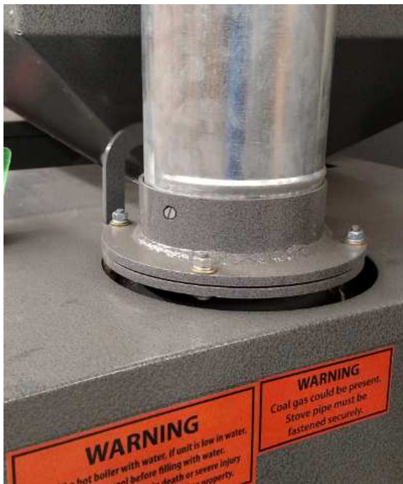
Flue Pipe Connection
