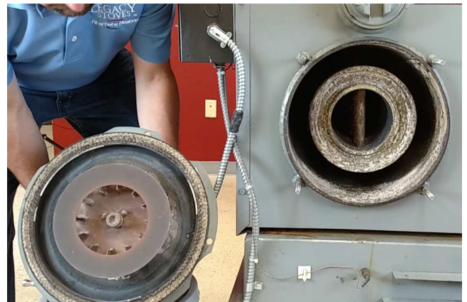
Set Aside Fan Assembly for Heat Exchanger Access
